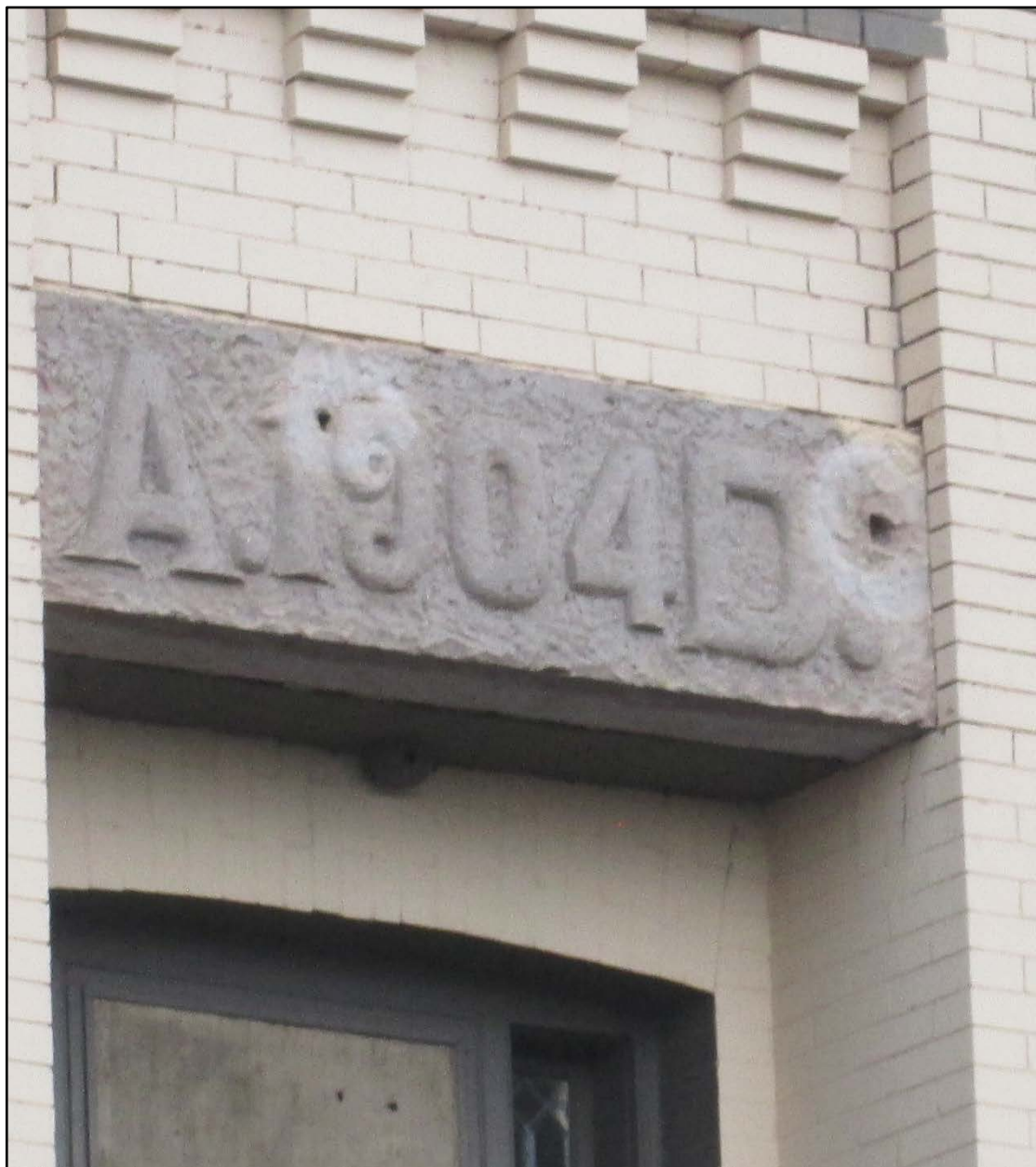
5PE575 – 112-114 W. 7th Street. Looking southwest at northern date plate above door. Photo ID: 5PE575g. June 2017.
