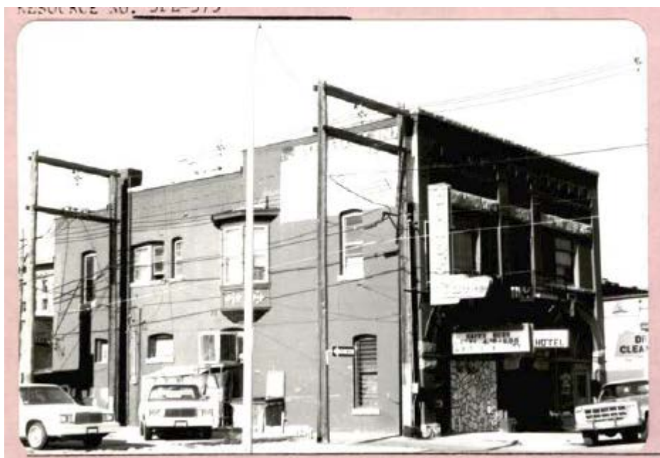
5PE575 – 112-114 W. 7th Street. Photograph from August 1981 recording.
