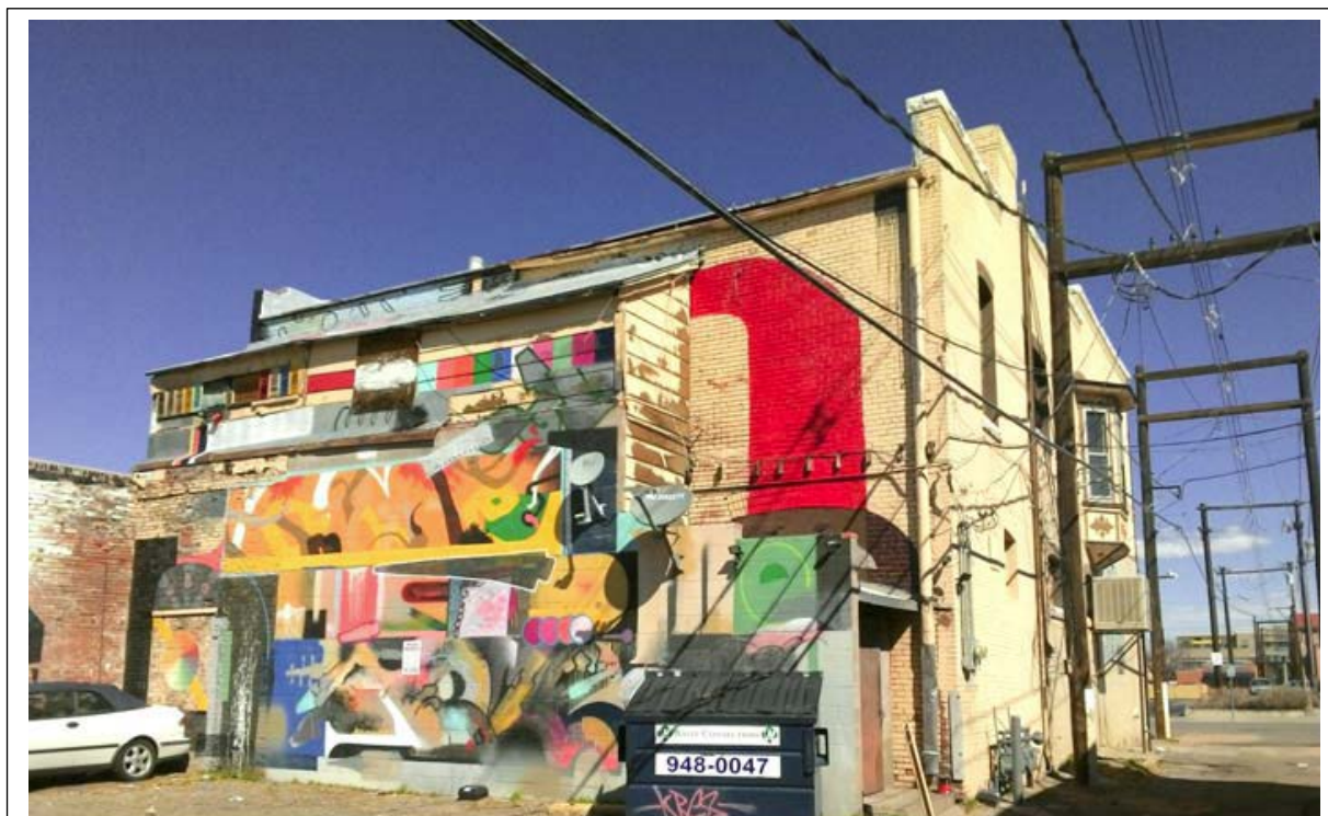
5PE575 – 112-114 W. 7th Street. Looking northwest at southern and eastern façades. Photo ID: 5PE575e. March 2016.
